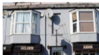
Bay windows opposite the site
