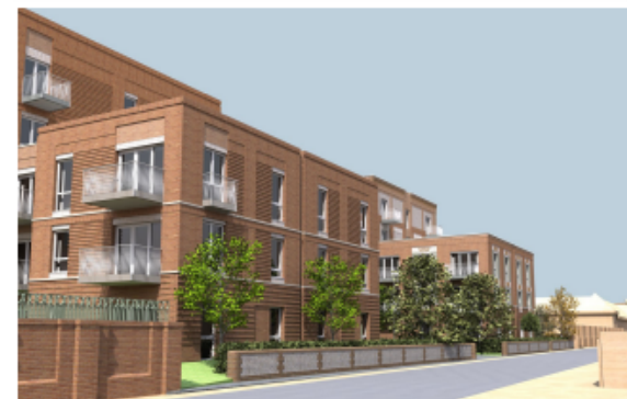
Lyndhurst Road looking towards the entrance
